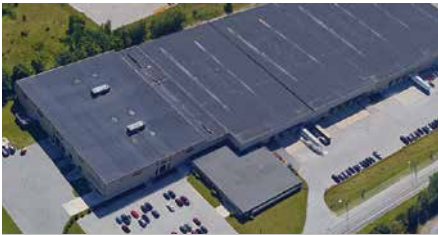
Barrie, ON (CAN) - High Performance Doors
